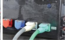
2. Insert the Cam connector into the receptacle and rotate Cam connector at least 90 clockwise degrees to lock
