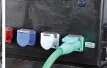
2. Insert the Cam connector into the receptacle and rotate Cam connector at least 90 clockwise degrees to lock
